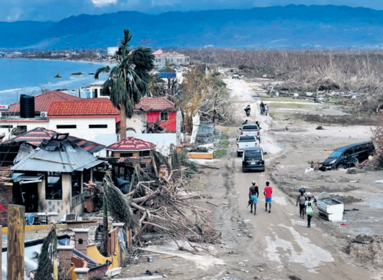
A drone view shows people walking in an affected area after Hurricane Melissa made landfall, in Crane Road, Black River, Jamaica, October 30
