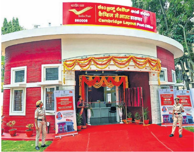
India's first 3D-printed post office is seen after its inauguration at the residential Cambridge Layout in Bangalore. The 3D-printed post office was built with a robotic printer using 3D printing technology that deposits concrete layer-by-layer in accordance with computerised 3D model drawing input
