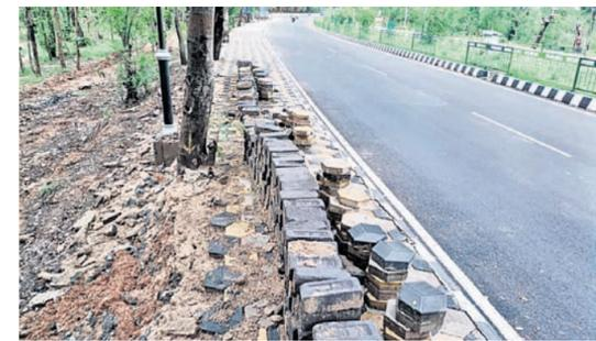
had been done wrongly. He pointed out that soil testing was not done in a proper manner before the laying of the blocks. "It takes at least two weeks for the soil to settle down after testing. However, it was not done and the paver blocks were laid in a hurried manner. Also no space has been provided for the rain-water to escape. Hence the paver blocks are collapsing," the retired official explained.
