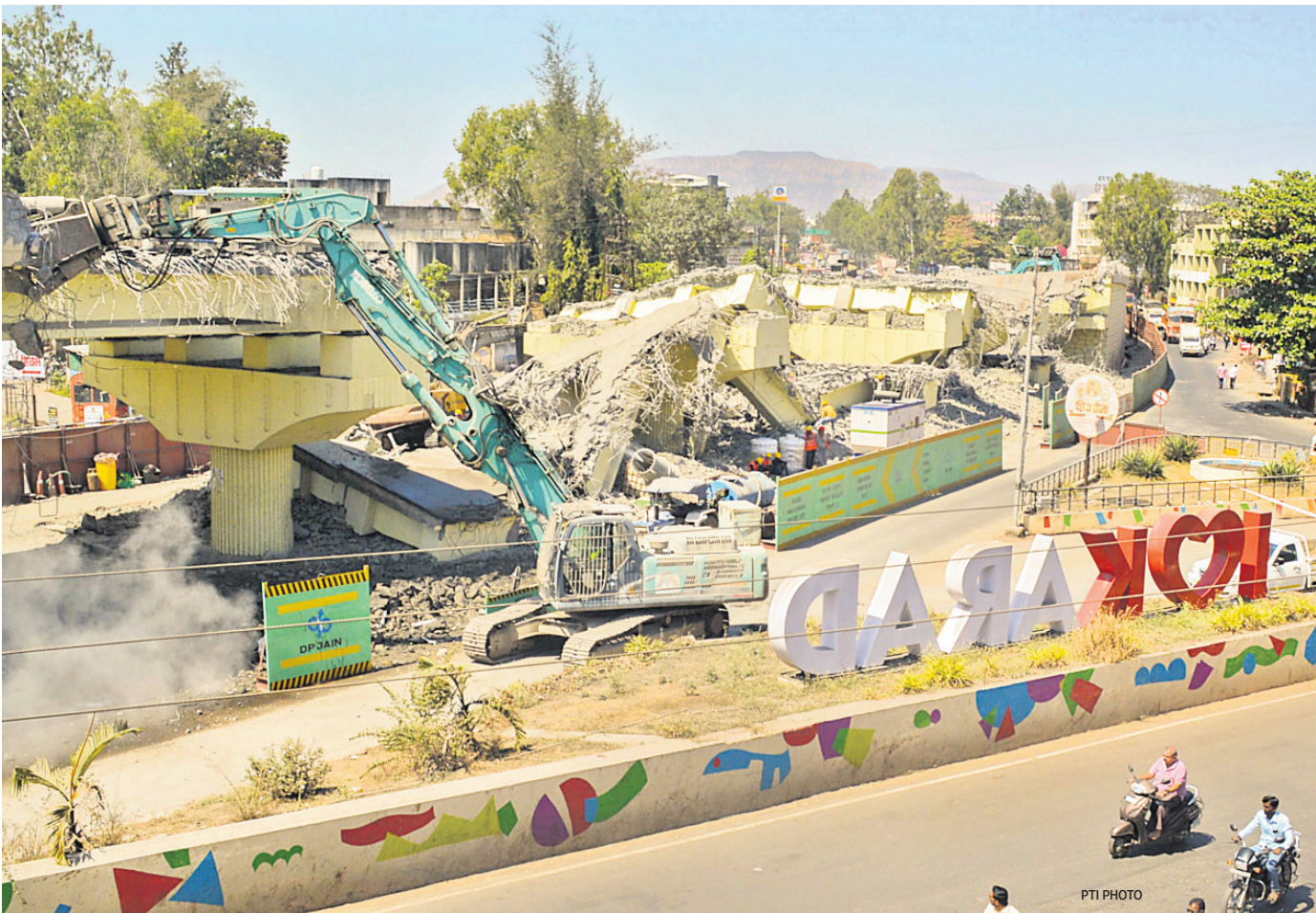
Kolhapur Naka Bridge being demolished as part of the six-lane work of Kagal-Satara stretch of Pune-Bangalore National Highway 48, in Karad, Maharashtra
