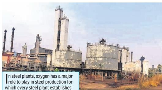
In steel plants, oxygen has a major role to play in steel production for which every steel plant establishes its own oxygen plant on its premises.
